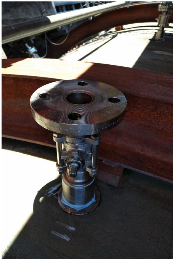
**Figure 2: Adapter and Valve Installed on the Original Acoustic Instrument Tap.**
