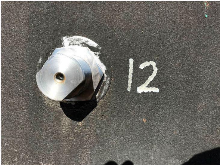
**Figure 1: Plugged Acoustic Instrument Penstock Tap.**
