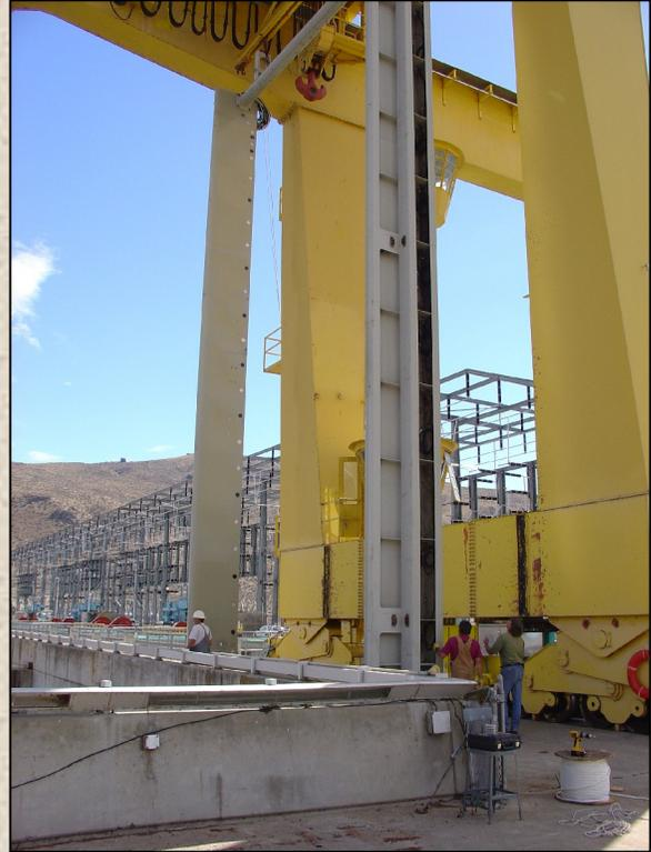
*ASFM Frame being lowered into intake*
