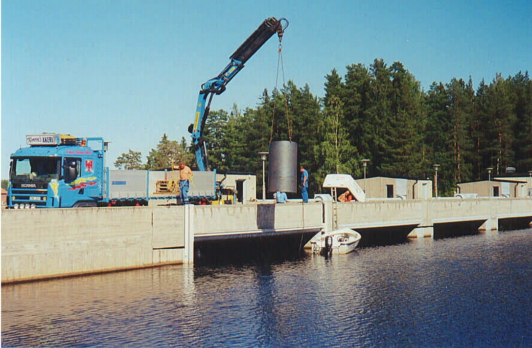
Figure 2-8: Transducer support frame fairings being installed prior to flow measurements.
