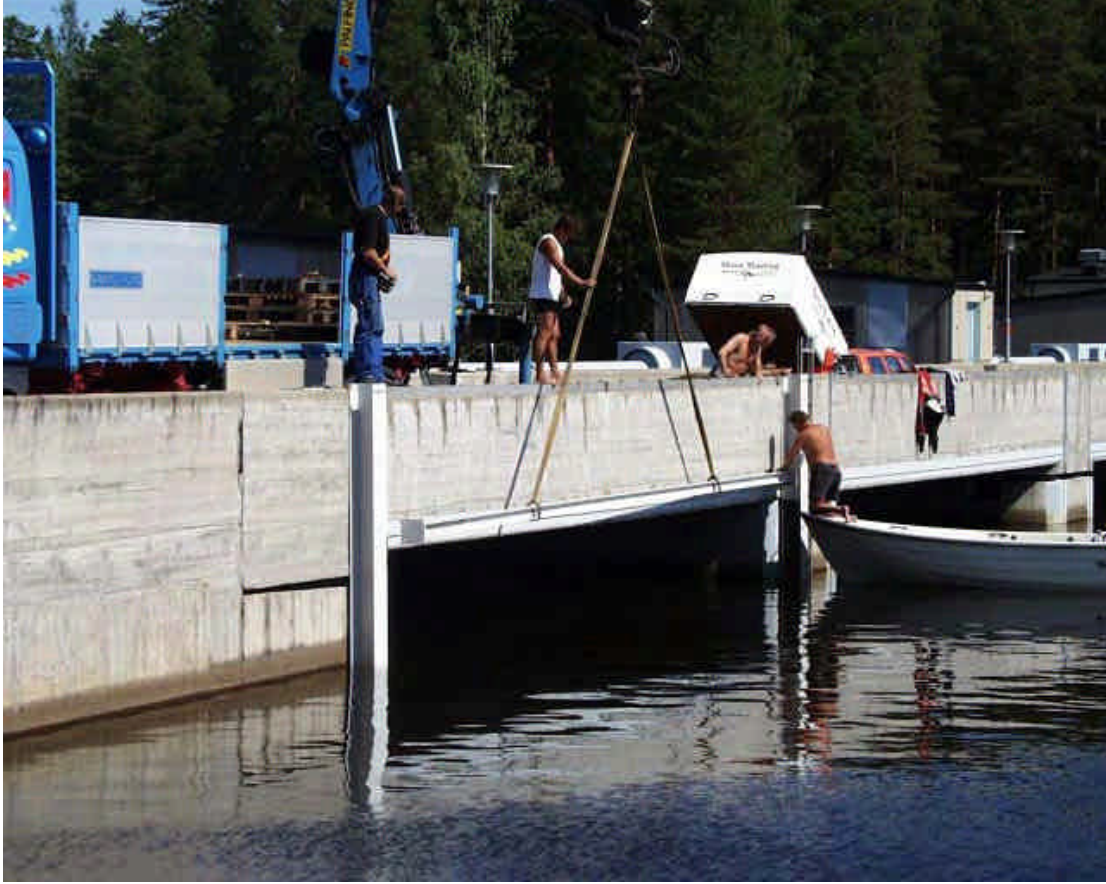
Figure 2-3: Transducer support frame being installed prior to vibration testing.
