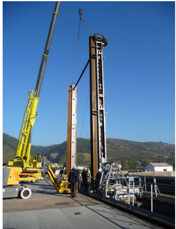
Figure 4: Picture of ADCP and ASFM frame
