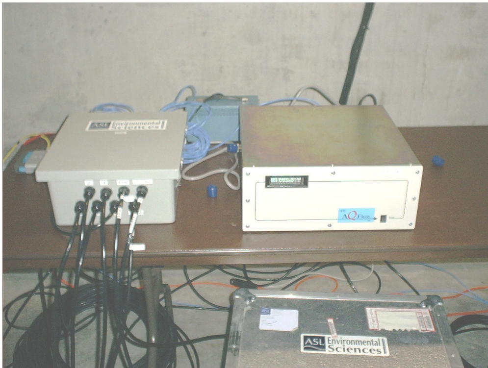
Figure 6: Monitor control unit and one switching box.
