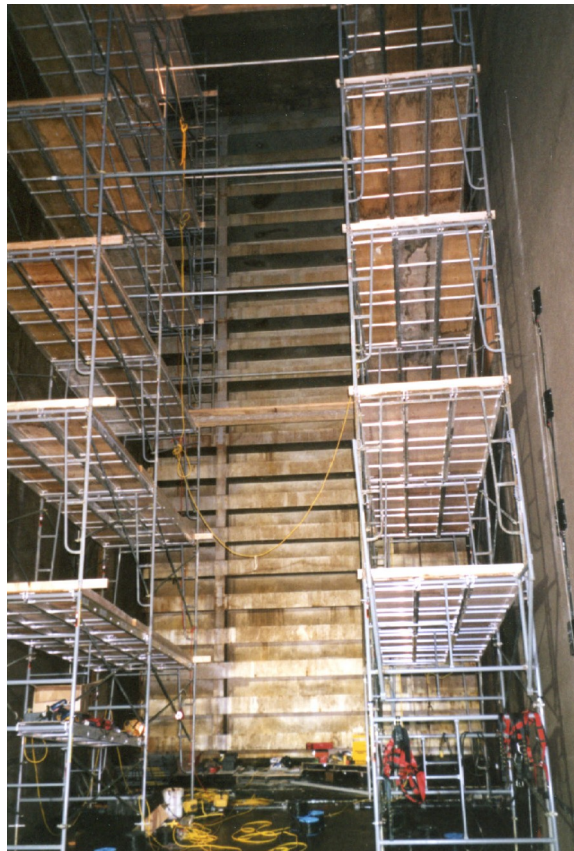
Figure 2: Interior of Bay A, Unit 4, during installation of the arrays and cabling.
