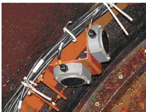
Fig. 5: Detail of transducer installation
