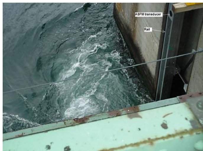
Figure 3 - Typical vortex in front of the ASFM transducer at Coteau-1
